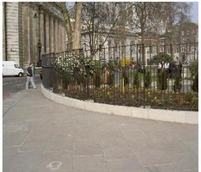
Stone kerb units around public park perimeter in conservation area. Non-standard kerb units to match existing profiles. All prepared to receive originals iron fencing in preformed leaded sockets, including supporting braces in T section units.
